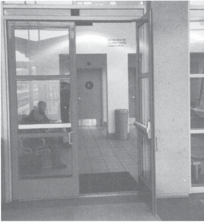
Fig. 3. Talking sign system above the door (black square) provides visually impaired people with a verbal message in a form that includes directionality.
